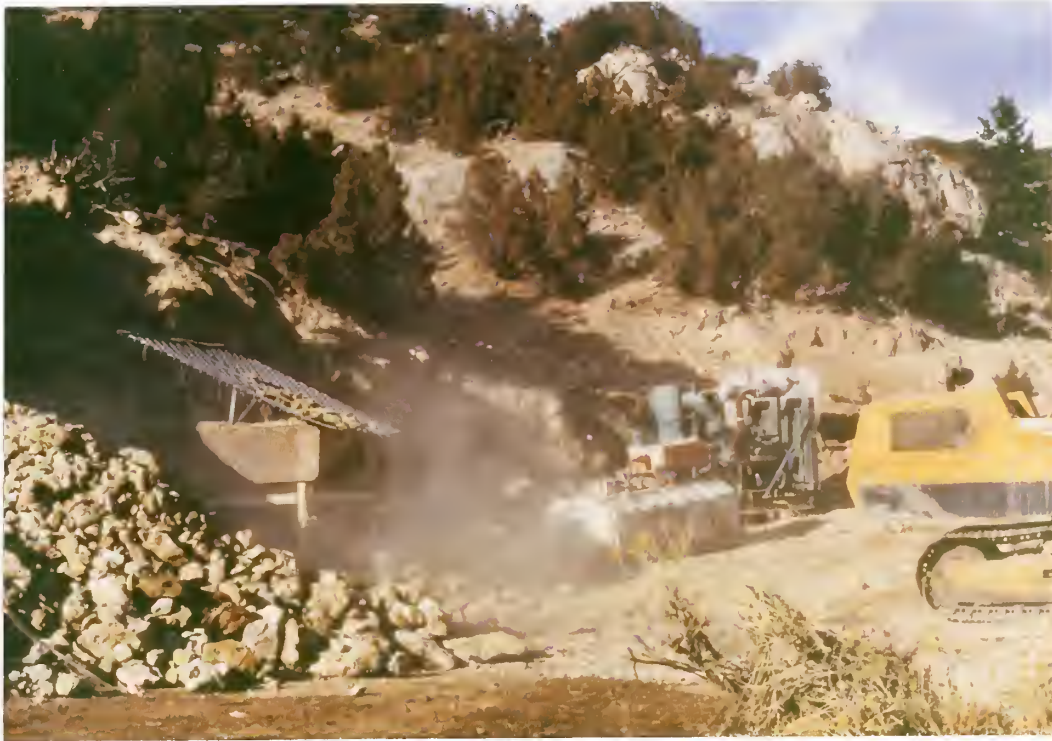
Typical Adit Backfilling Using Conventional Machinery To Feed Pneumatic Injection Equipment
